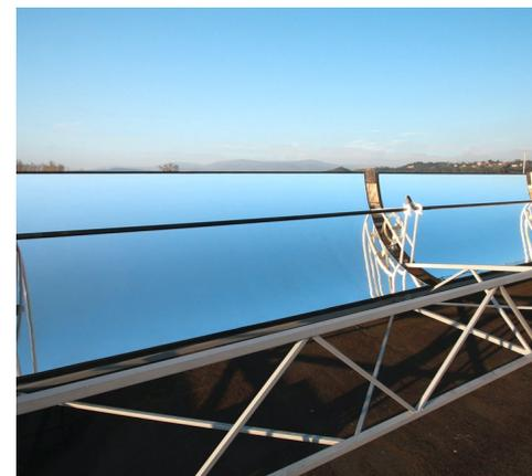
Prototypes of Helioclim solar panels on roofs
